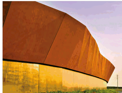
QB42 Craigieburn Bypass, Melbourne High quality integrated noise and retaining walls with articulated surfaces
