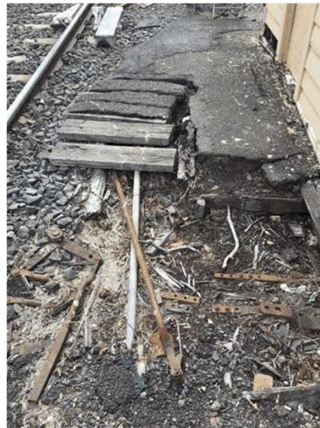
2019, Remnant interlocking equipment outside signal box.
